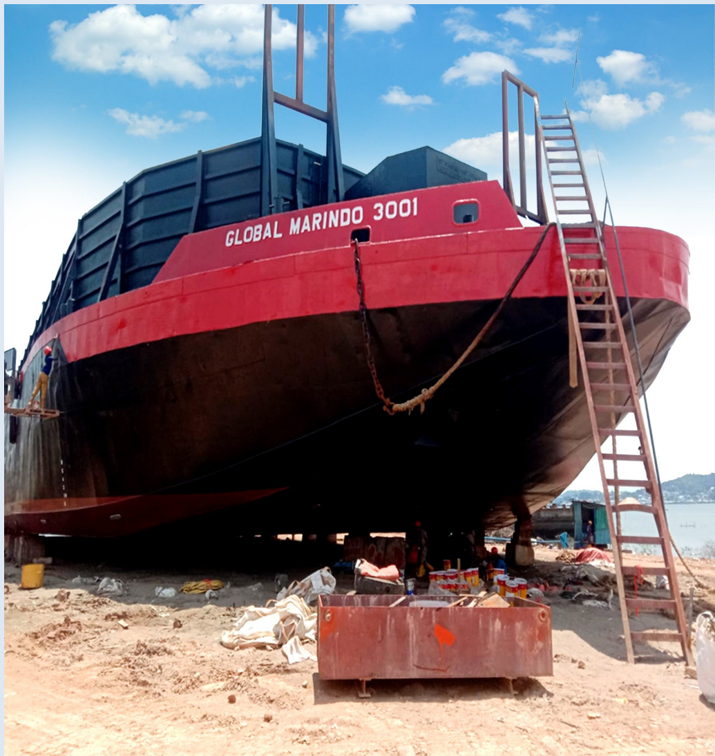
BARGE REPAIR BARGE NAME : GLOBAL MARINDO 3001
